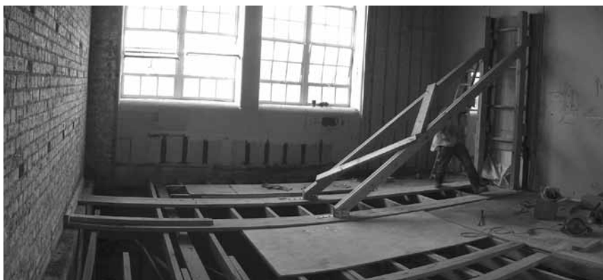
Figure 11. Reaction frame constructed for out-of-plane testing
