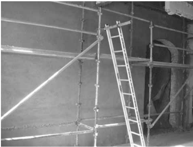
Figure 19. W1 after shotcreting
