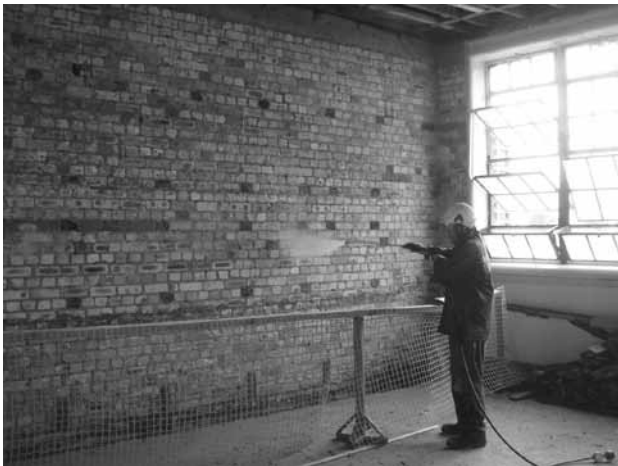
Figure 16. Water-blasting of masonry surface to prepare for shotcrete
