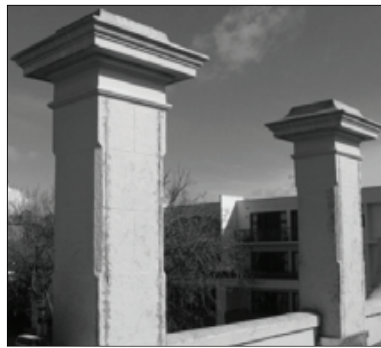
(b) Rear chimneys retrofitted using NSM CFP
