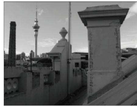
(c) Chimneys retrofitted using NSM CFP
