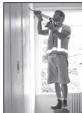
(c) Epoxy application
