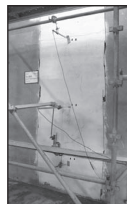
(c) Typical instrumentation setup (Allen's Trade Complex)
