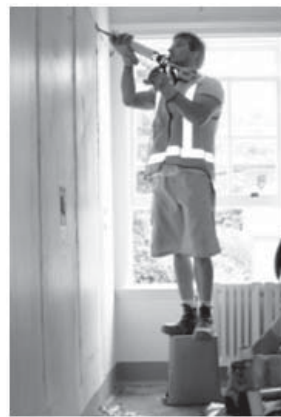
(c) Epoxy application
