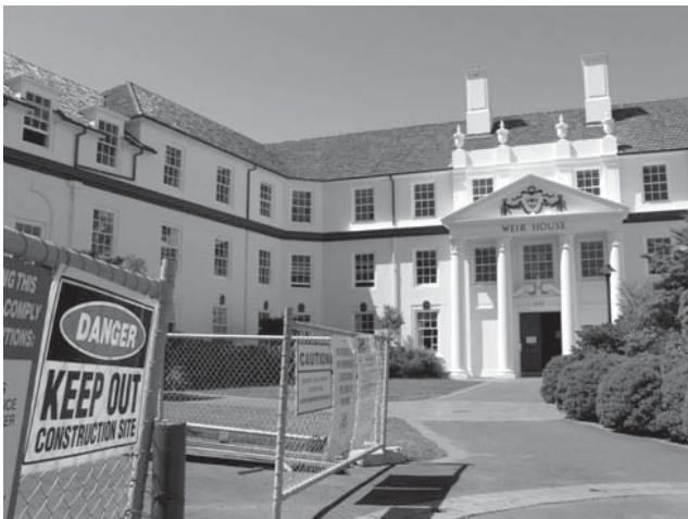
(a) Street view (facing S-E)
