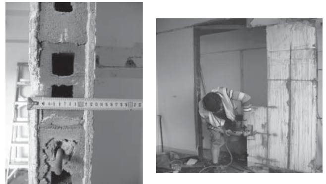
(a) Partition wall cross section (b) Masonry prism extraction
