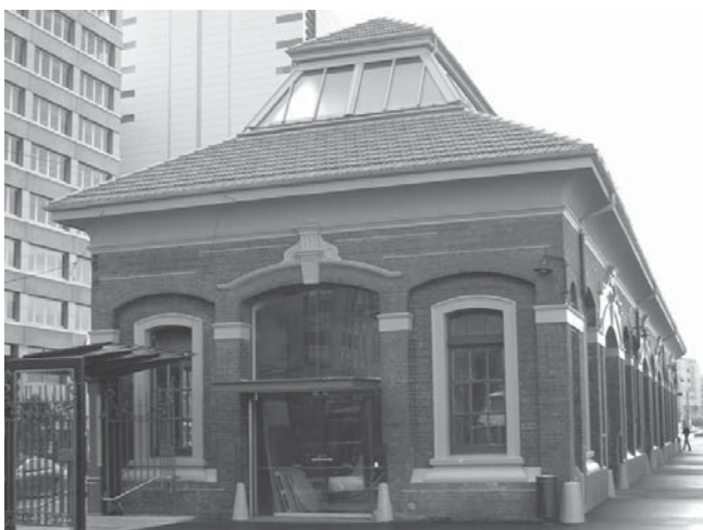
Figure 6. Shed 13 on the Wellington waterfront, that features a distinctive roof that is integral with its character
