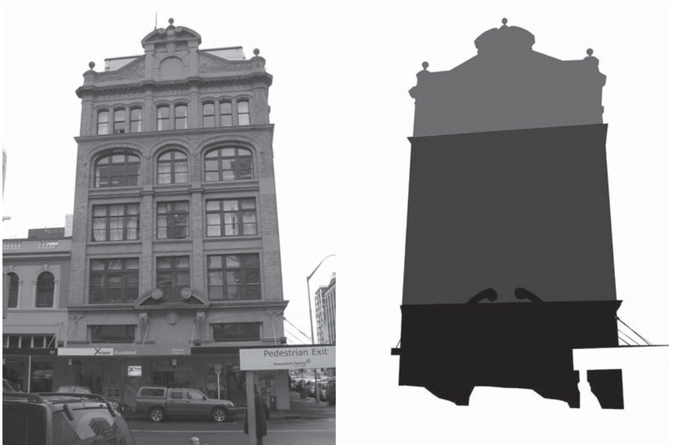
Figure 4. Primary form of a URM building in Auckland. At this stage the basic shape and the broad gestures that make up the building are noted. In this case the building has a reasonably simple form and displays a typical 3 part vertical hierarchy
