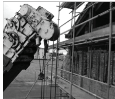
(c) Lifting wall panels using a medium sized crane
