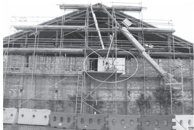
Figure 9. In-plane push test location, southern gable
