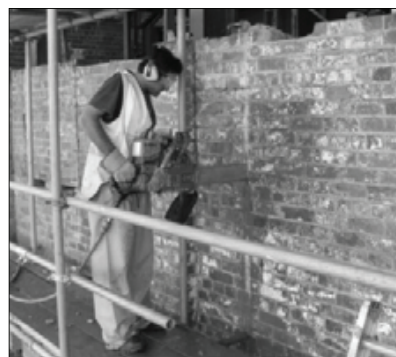
(a) Cutting through masonry
