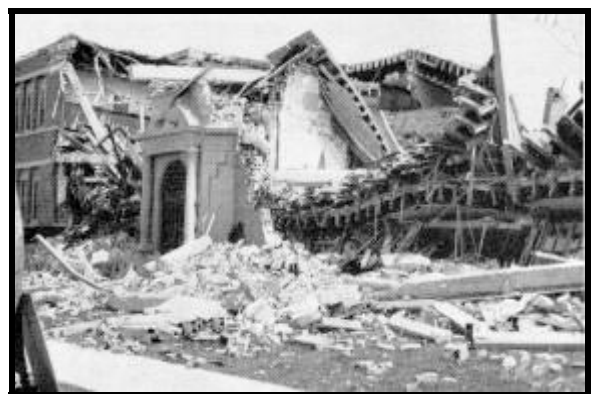
Figure 2 The collapse of part of Jefferson Junior High School in Long Beach 1933 (reproduced from [31])
