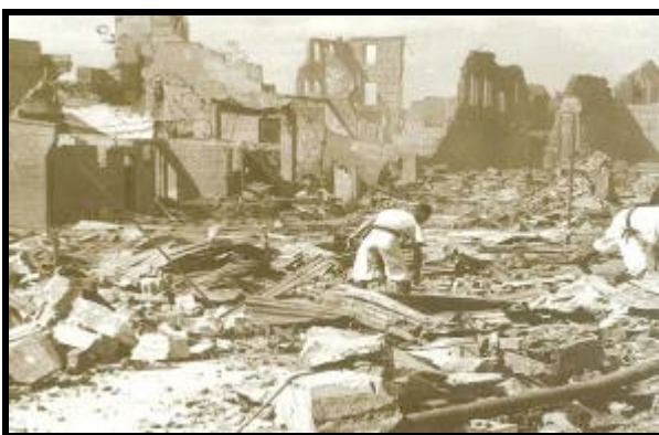
Figure 1 Damage to URM buildings in Napier earthquake 1931 (reproduced from [30])
