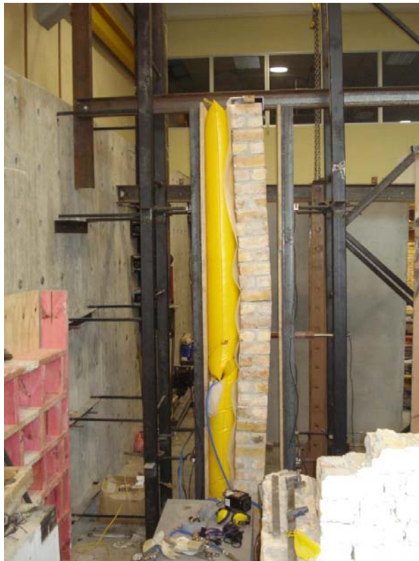
Figure 2: A single horizontal crack began to develop 350 mm above the wall mid-height; the supports at top and bottom of the wall allow for rotation of the wall, and therefore no crack was formed at the support levels. Four load cells connecting the backing frame to reaction frame at each side, and the single LVDT arrangement can be observed in the figure.
